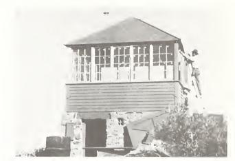
Figure 44. St. Peters Dome lookout house (L-4), Santa Fe National Forest, New Mexico, photographed in 1946 during repair work on the windows. It was constructed between 1933 and 1935 (U.S. Forest Service photo).
